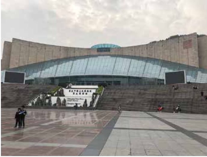
Photo 8.25 The magnificent façade and entrance to the Three Gorges Museum, Chongqing
