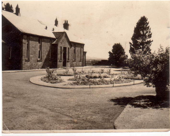
Figure 1.19 One of the two wards at Strathmore Hospital in Blairgowrie.
